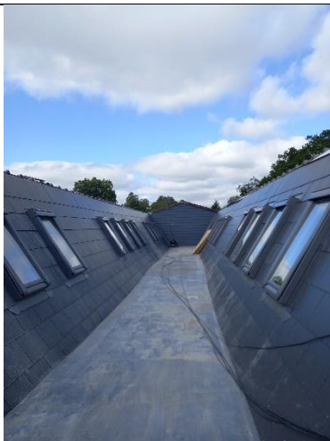
Photograph 5 - HSC Block - New Velux installations and artificial slates
