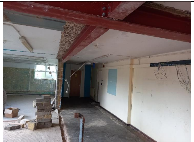
Photograph 6 - MFL toilets reconfiguration Steel installed.
