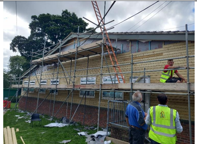
Photograph 4: Cladding installation complete to North Elevation.
