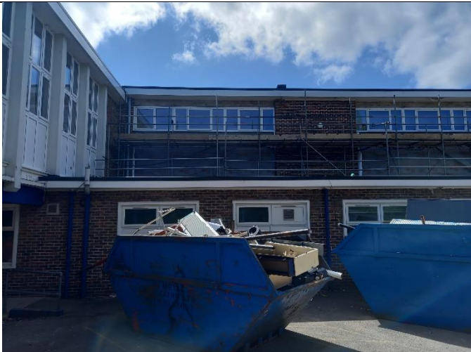
Photograph 3: English block, Asbestos containing cladding removal commenced.
