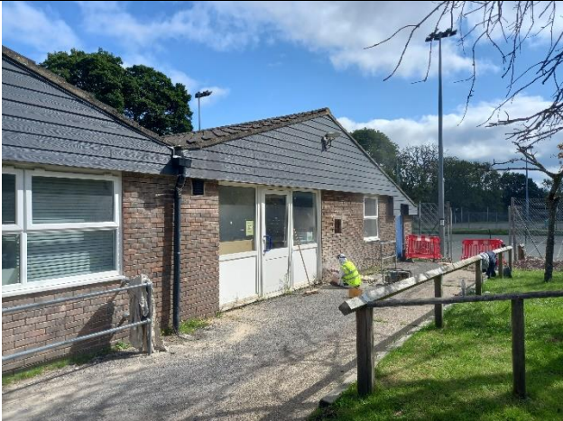
Photograph 1: Brickwork repairs on-going to Art Block.
