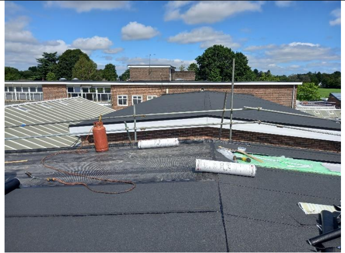
Photograph 2: Roof 7 - Works nearing completion.
