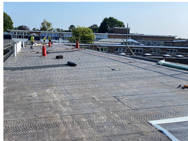
Ongoing renewal of roof coverings
